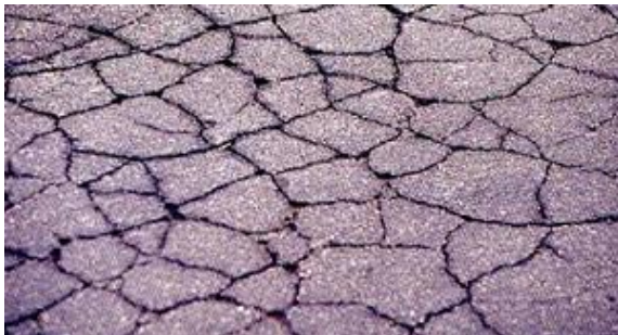
Figure 1. Growth of fatigue cracks caused by applied traffic load on asphalt pavement
