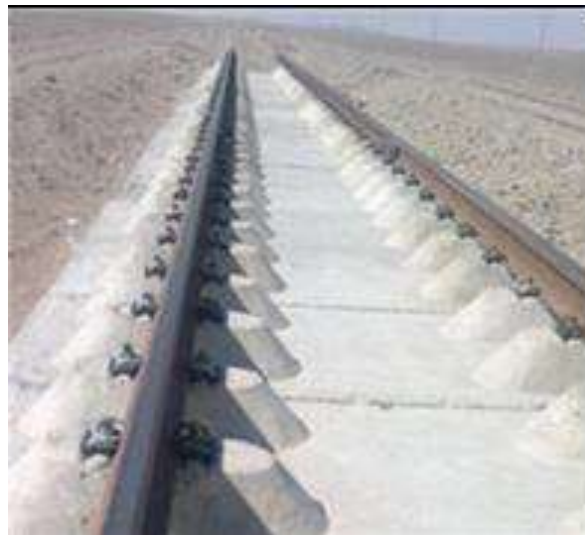
Figure 4. Dumped slab track design
