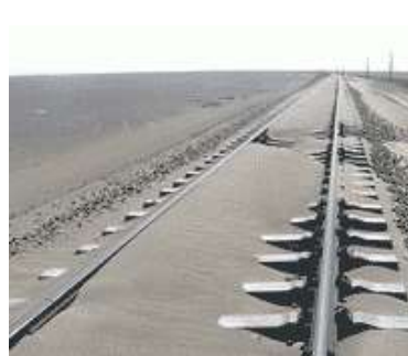
Figure 1. Entry of sand into railway track, burial of track under sands, and inefficiency
