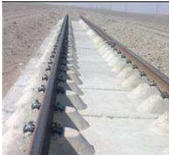
Figure 4. Dumped slab track design
