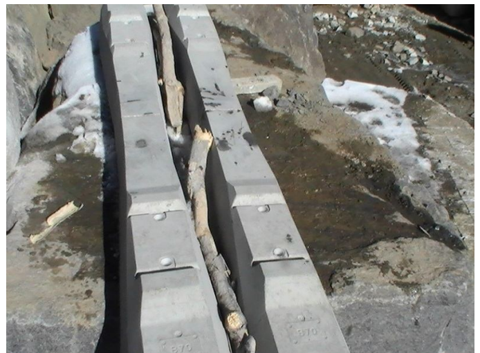
b. Center notched sleepers.
